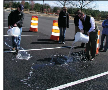
Porous parking lot at Johnson & Johnson Pharmaceutical Research and Development campus
