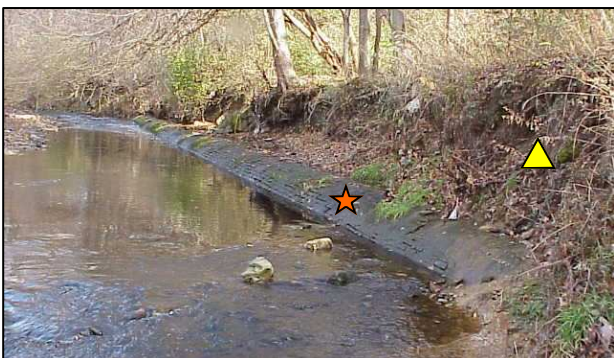
The creek at Marshall Road suffered from severely eroded banks ( triangle ) and exposed infrastructure ( star ).
