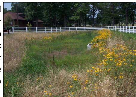
Naturalized stormwater detention basin at Black Rock in Upper Providence Township
